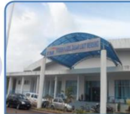
Cable Landing Station
